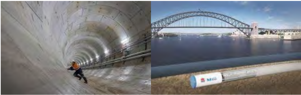
The Sydney Harbour Tunnel construction and visual map
