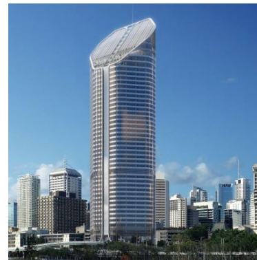
1 William Street, located in the heart of Brisbane City, will become its largest commercial building upon completion.
